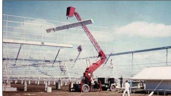
Figure 7: Closing the Cross. The East 1 feed is lifted off the telescope near midday on 24 August 1978.
