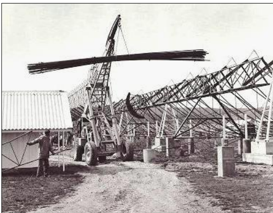
Figure 4: Erection of the East arm reaches the centre. The insulated phasing hut is on the left.
